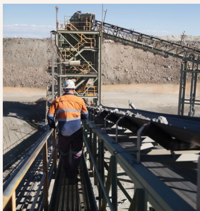
Tritton ore transfer conveyor
