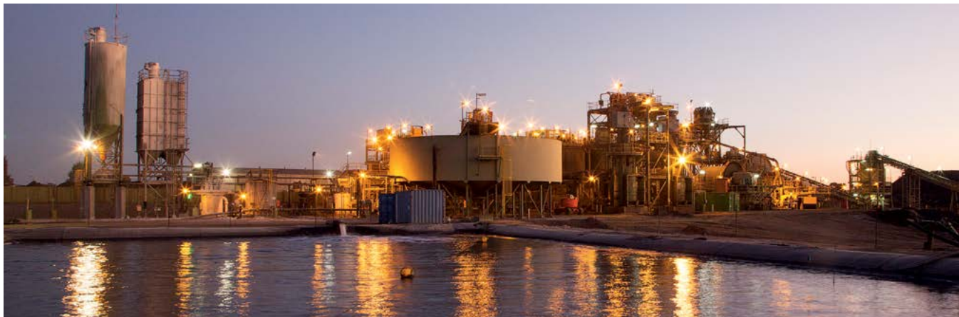
The processing plant at Straits' Tritton operations
