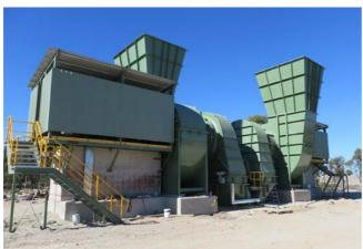
Figure 2: Ventilation Fans installed at Tritton Underground Mine over the new exhaust ventilation shaft
