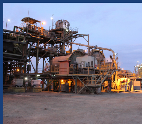
Aeris Resources Tritton Copper operations in NSW.
