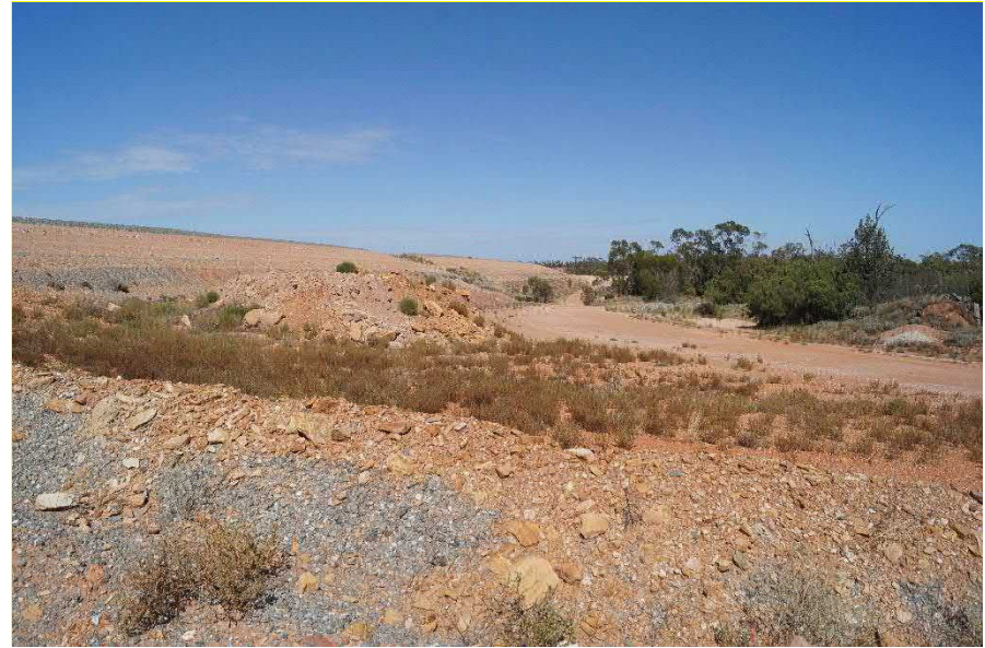
North wall with spillway – looking west (17/2/2022)
