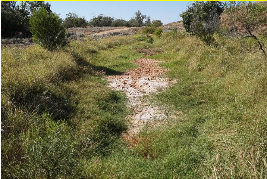
View looking south along downstream toe drain (17/2/2022)
