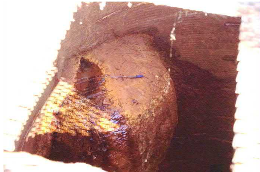
Underdrainage water flowing into sump for return to the process plant (17/2/2022)
