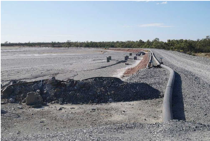
Western embankment-decant access intersection - looking south (17/2/2022)
