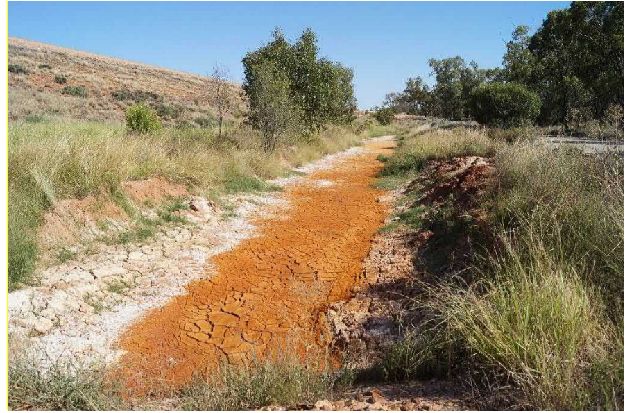
View looking north along downstream toe drain (17/2/2022)
