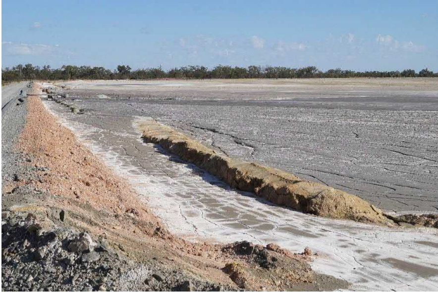
Western embankment-decant access intersection - looking north (17/2/2022)
