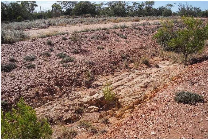
Bedrock exposed at toe of east wall of TD1 (17/2/2022)
