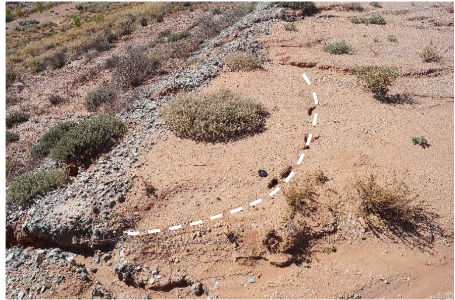
Incipient slumping of the east wall intermediate berm crest (17/2/2022)
