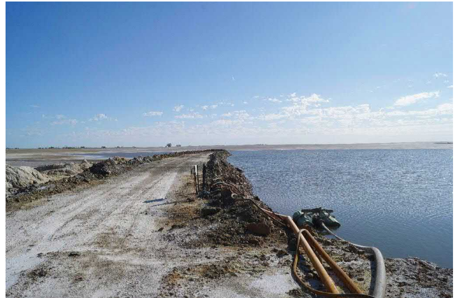
View along decant access roadway - looking east (17/2/2022)
