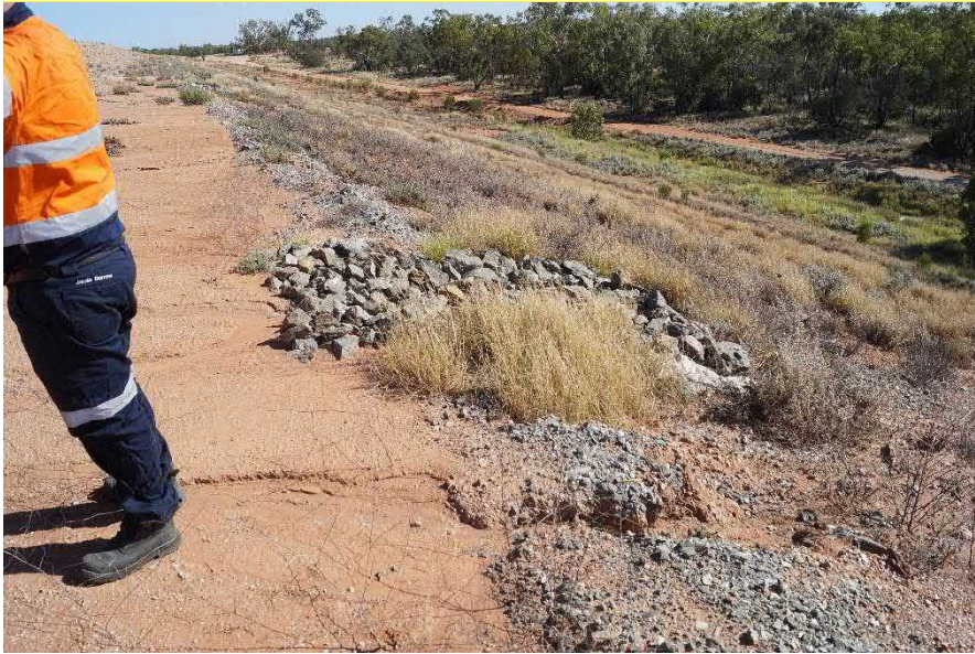
Rip-rap channel on east wall of TD1 - looking north (17/2/2022)
