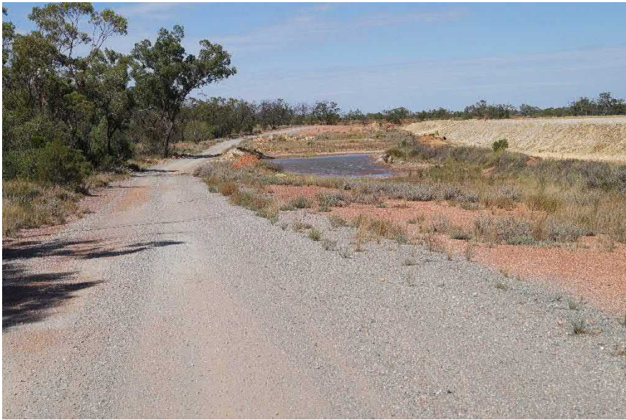
Interception dam south of TD1 (17/2/2022)
