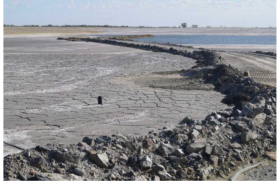
Decant access roadway - looking east (17/2/2022)
