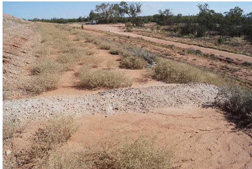
Cut-off bund on intermediate berm on east wall - looking north (17/2/2022)
