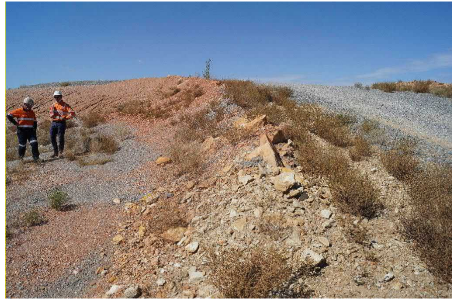
Construction access ramp at north end of main east wall (17/2/2022)
