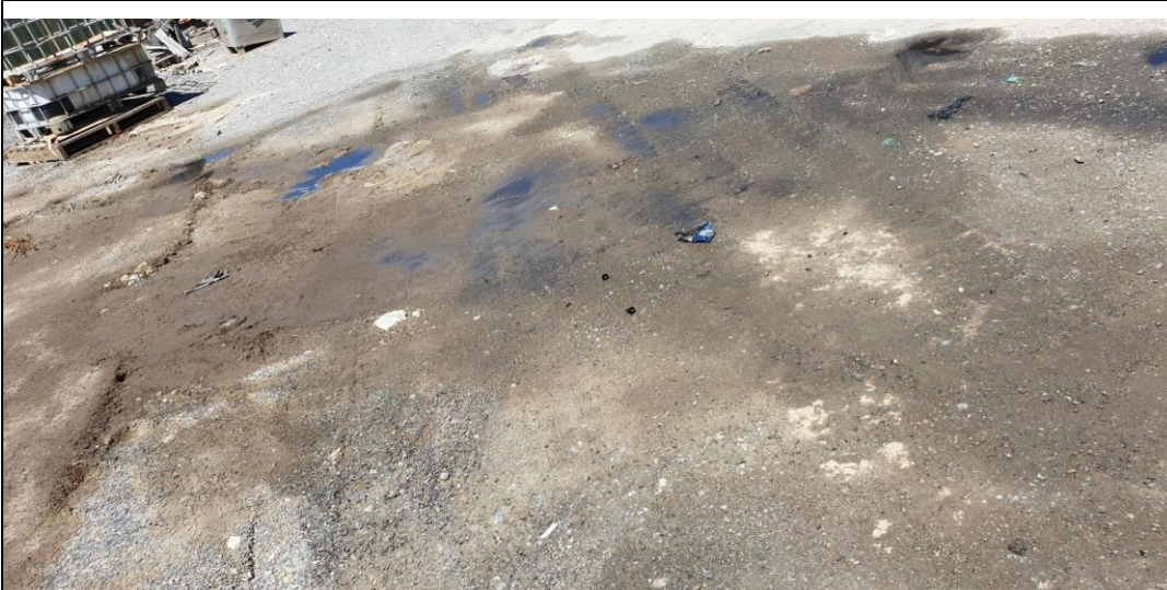
Photo 12: Surface pollution from recent material movement, not managed (NC 19)
