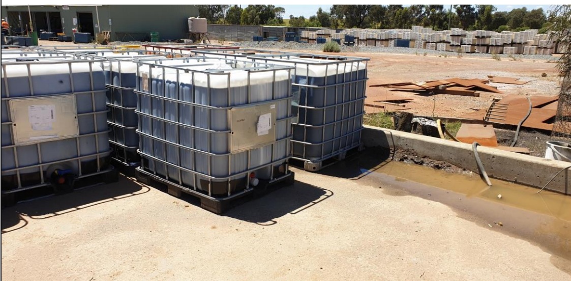
Photo 8: Container storage area near workshop, with inoperable drain pump-out system (NC 19)
