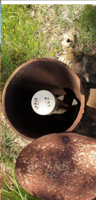
Photo 2: Groundwater monitoring well
