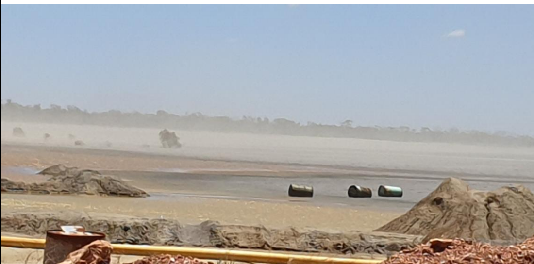
Photo 10: Dust emission from TSF surface
