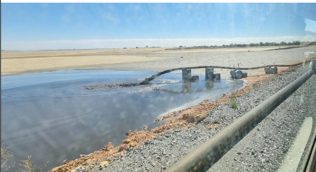
Photos 16 and 17: TSF pump in system
