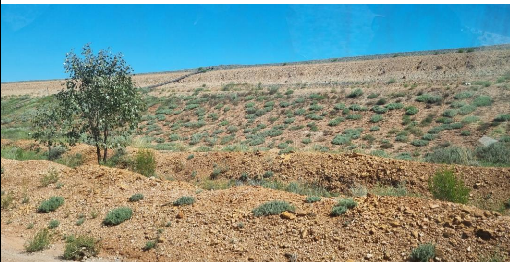
Photo 20: Rehabilitation on TSF embankment wall
