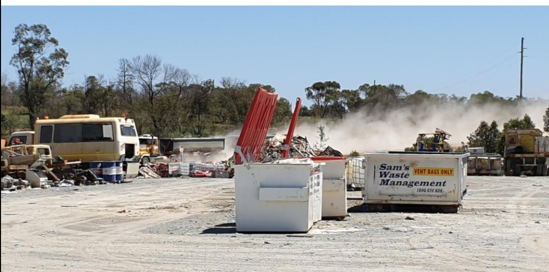
Photo 11: Dust emission during heavy vehicle operation – no water cart was in operation (NC 1)
