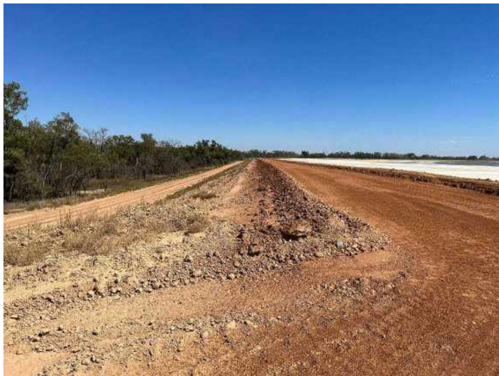
View along the western embankment looking north.
