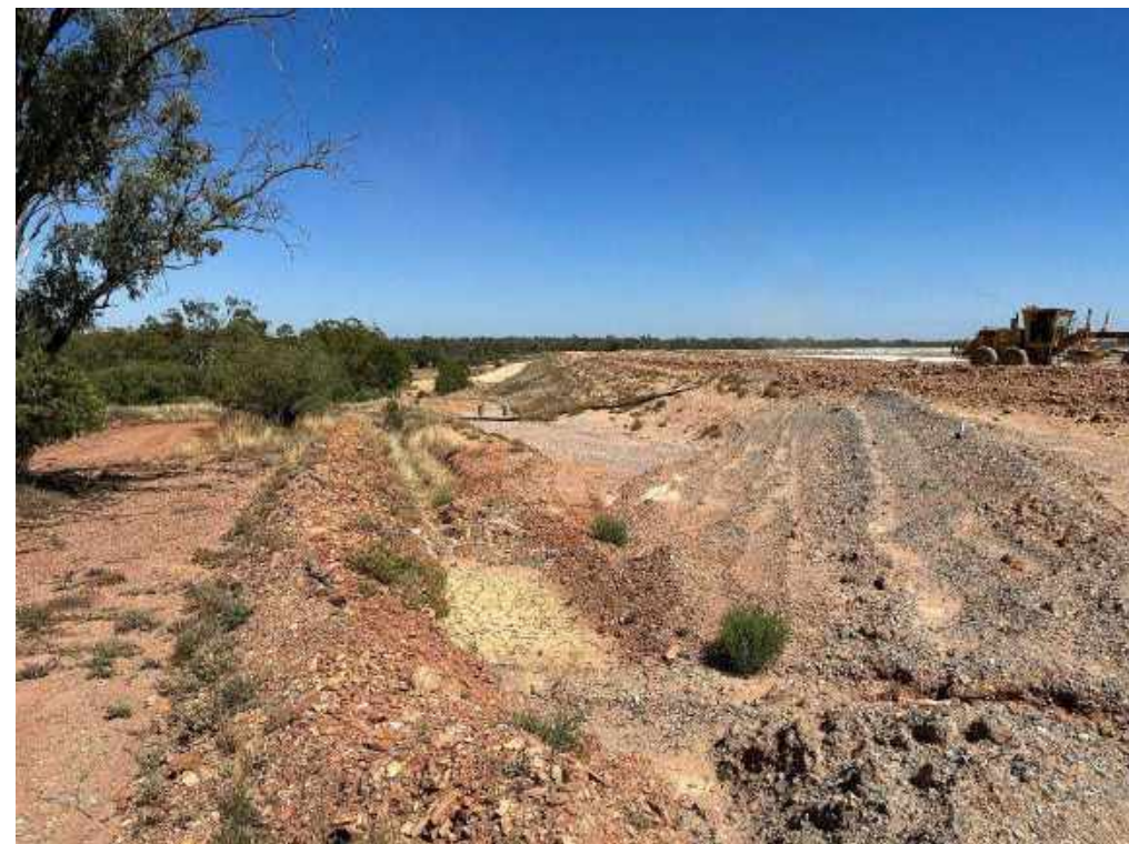
View along south western side of TD1, downstream looking north west.
