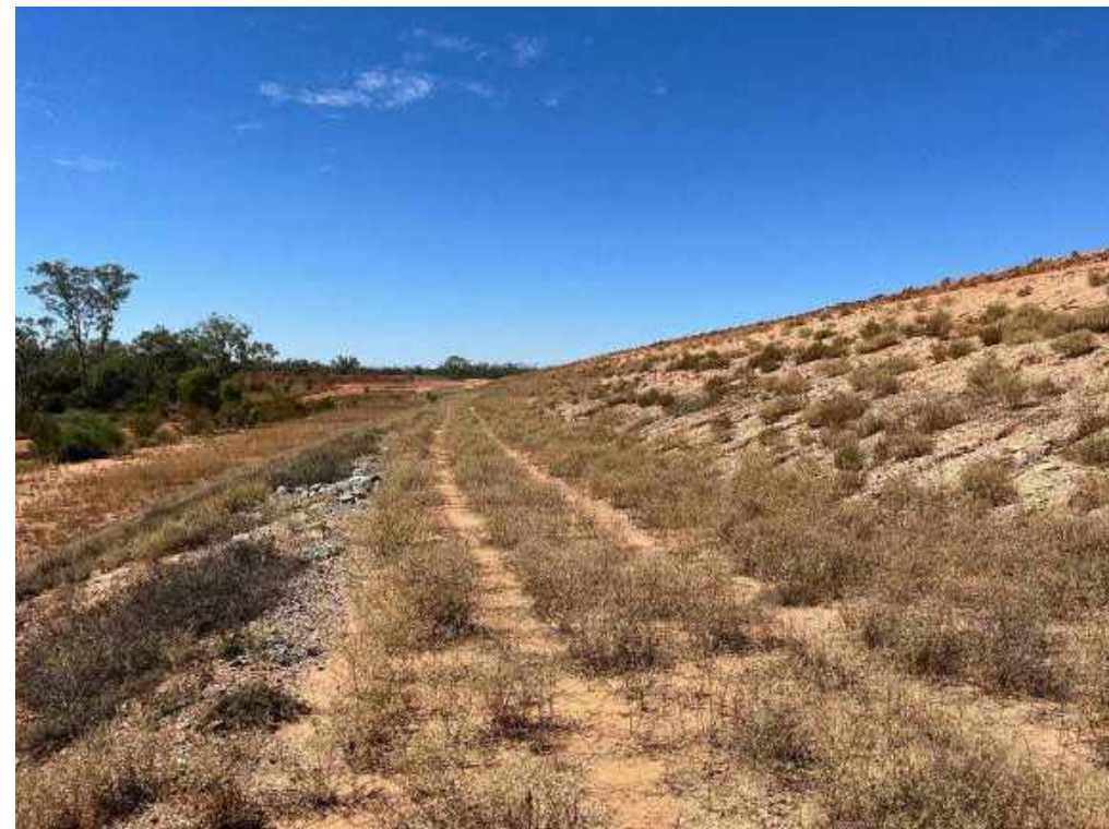
View of Main Embankment southern end looking south.
