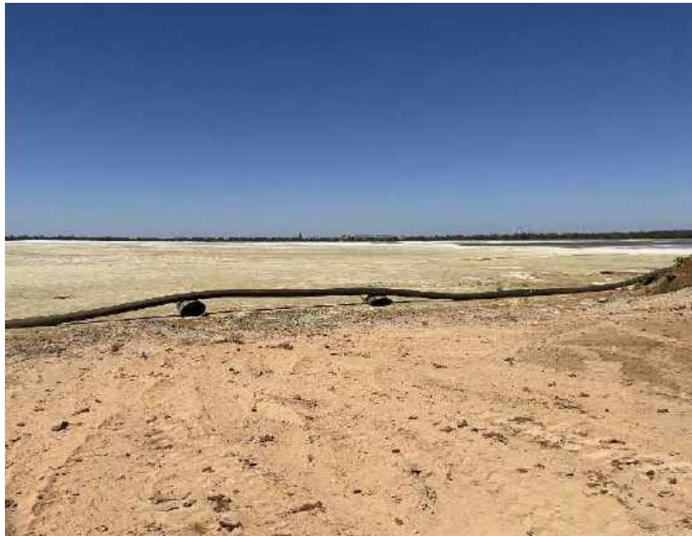
Spillway entrance looking to the decant.
