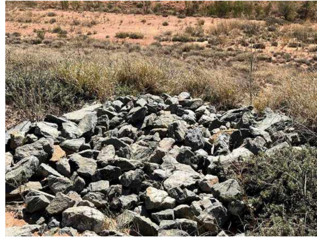
Typical erosion repair at intermediate berm, northern end.
