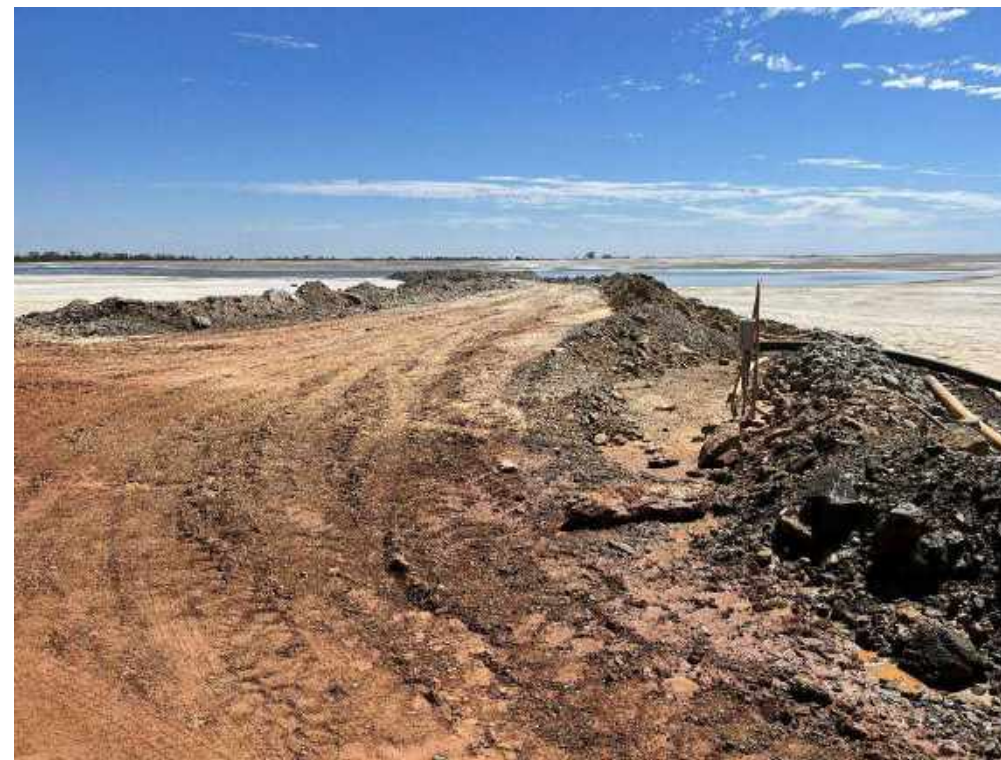
Panorama from western embankment looking east.
