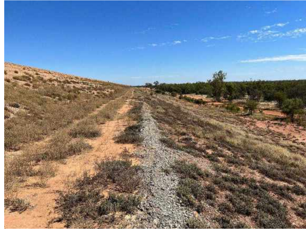
View of Main Embankment southern end looking north.
