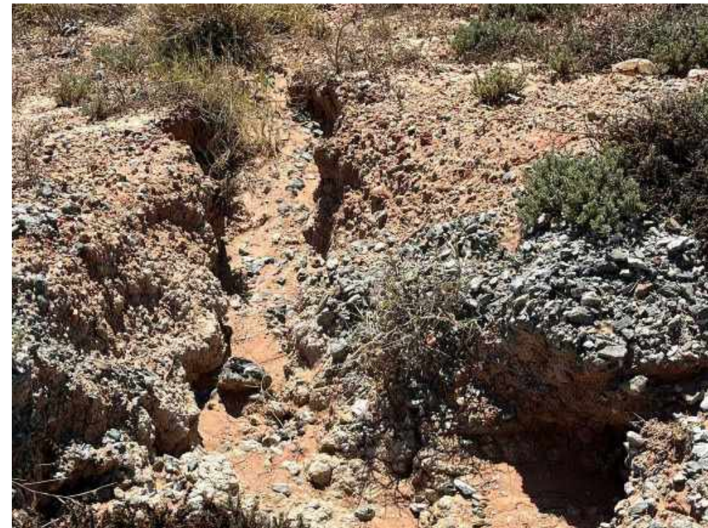
View of collapsed piping hole intermediate berm, northern end.
