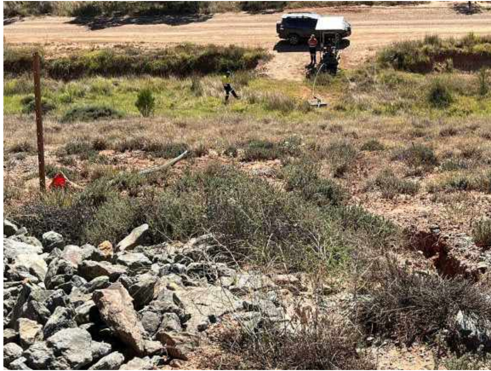
View of erosion repair and gully erosion upslope of underdrainage sump.
