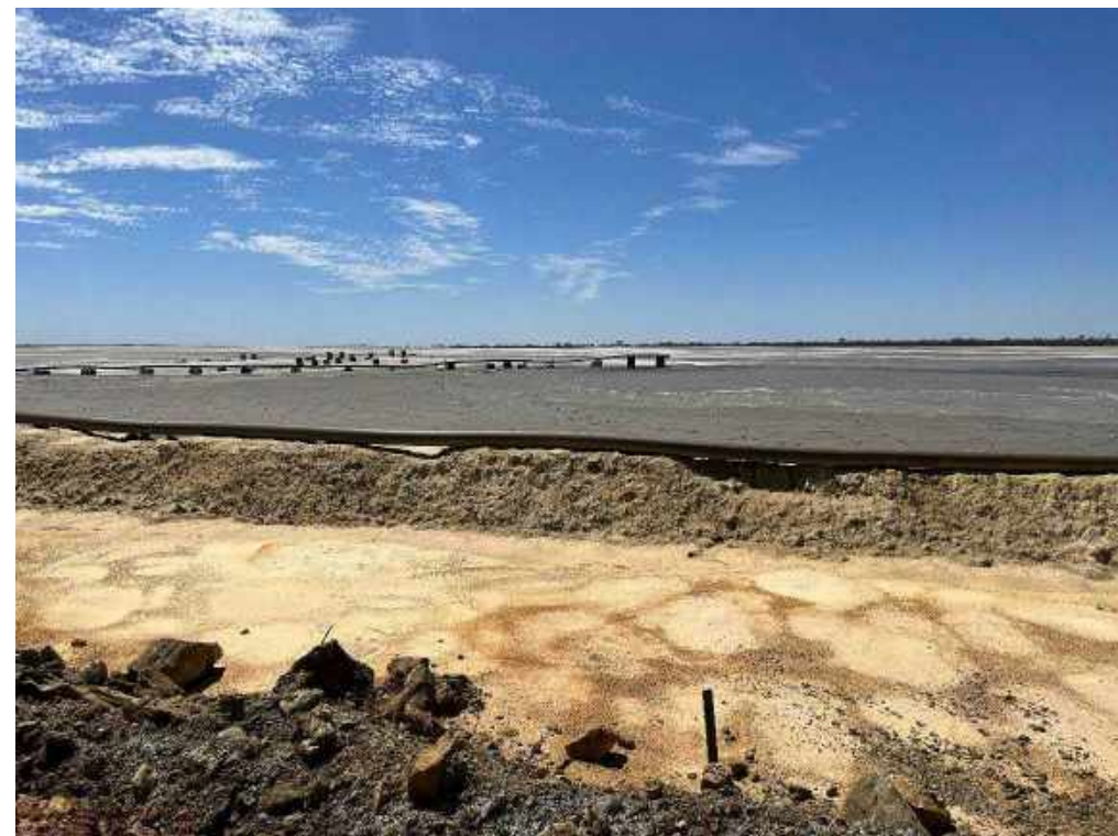
View of recent tailings slurry discharge northern side of TD1.
