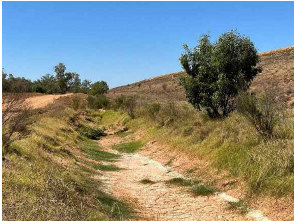
View looking south from sump, along main embankment toe.
