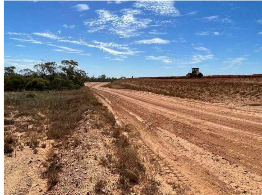
View of embankment raising works northern side of TD1, from downstream.
