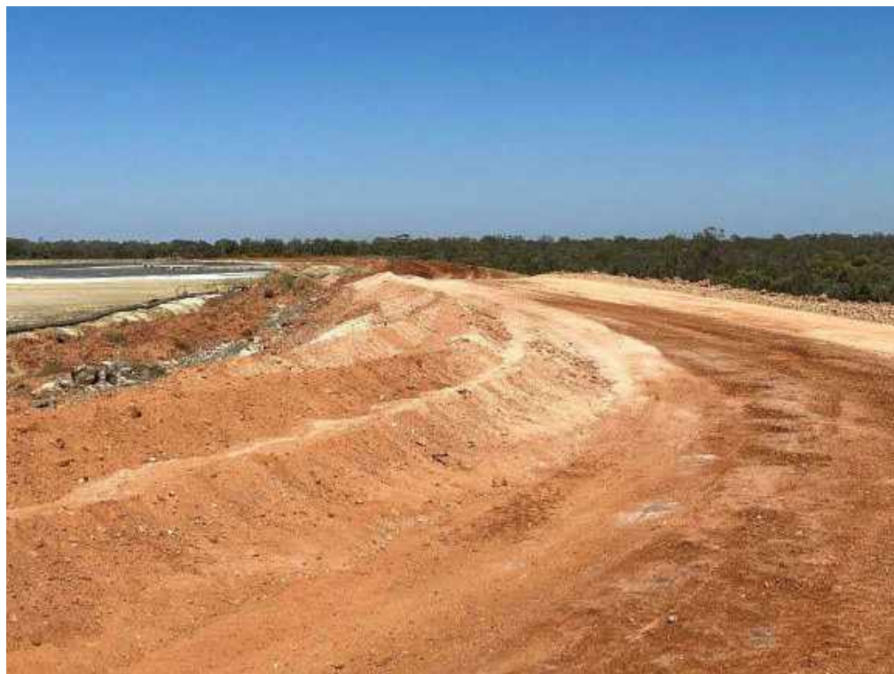
View along northern embankments, upstream looking west.
