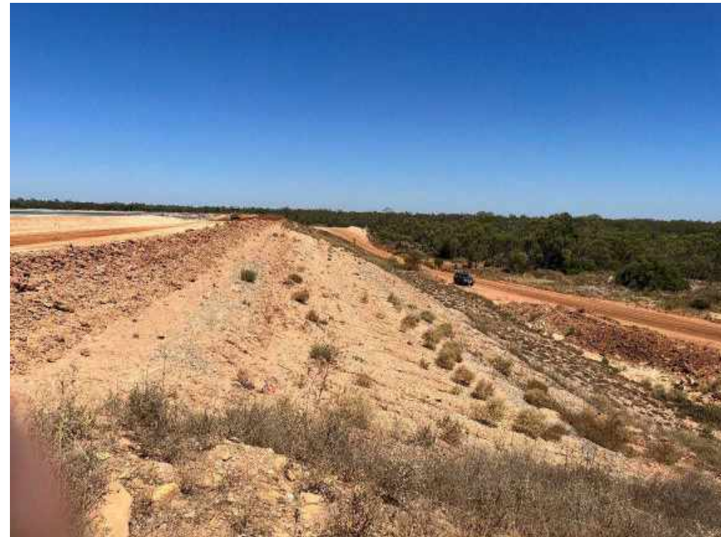
View of embankment raising works northern side of TD1, looking west.
