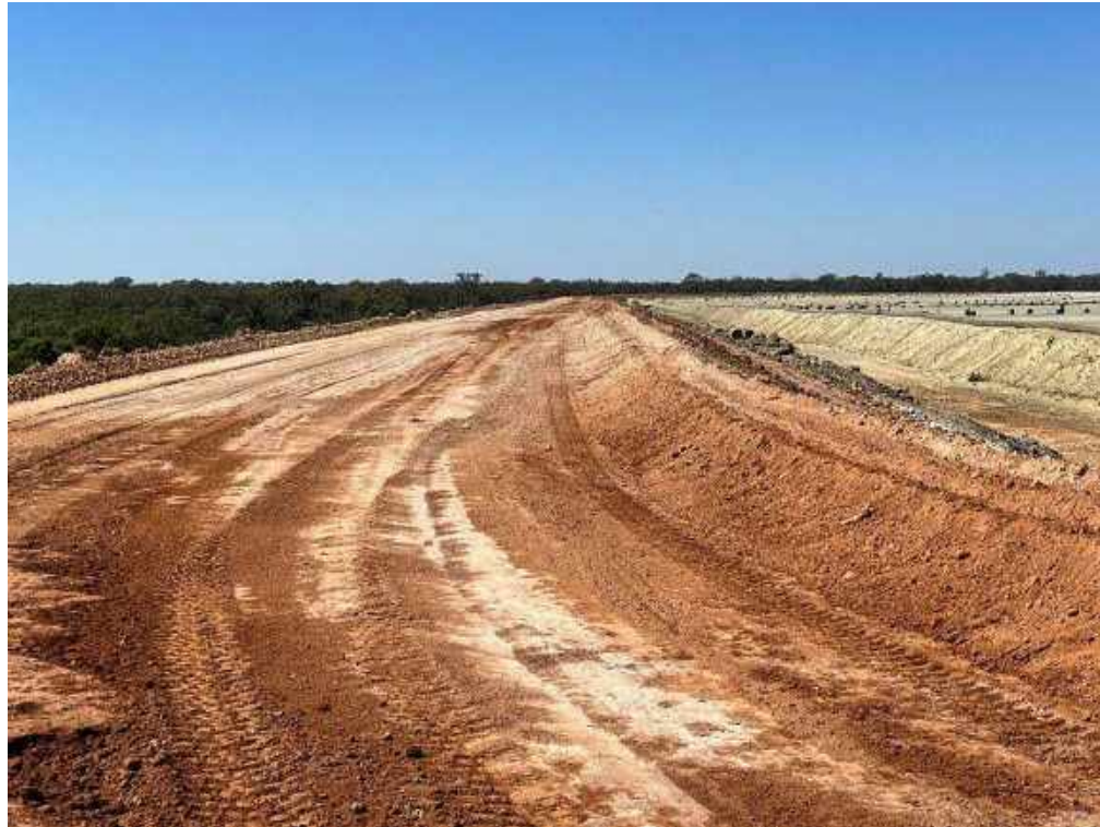
View along main embankment, upstream looking south.
