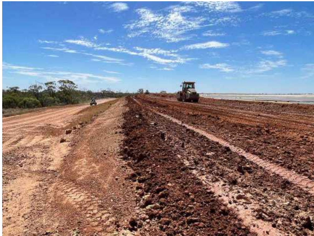
View of embankment raising works northern side of TD1.
