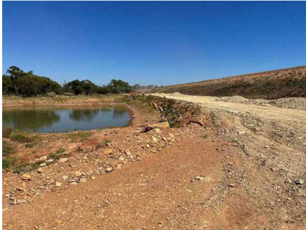
View of pond and pump, adjacent south western embankment of TD1.
