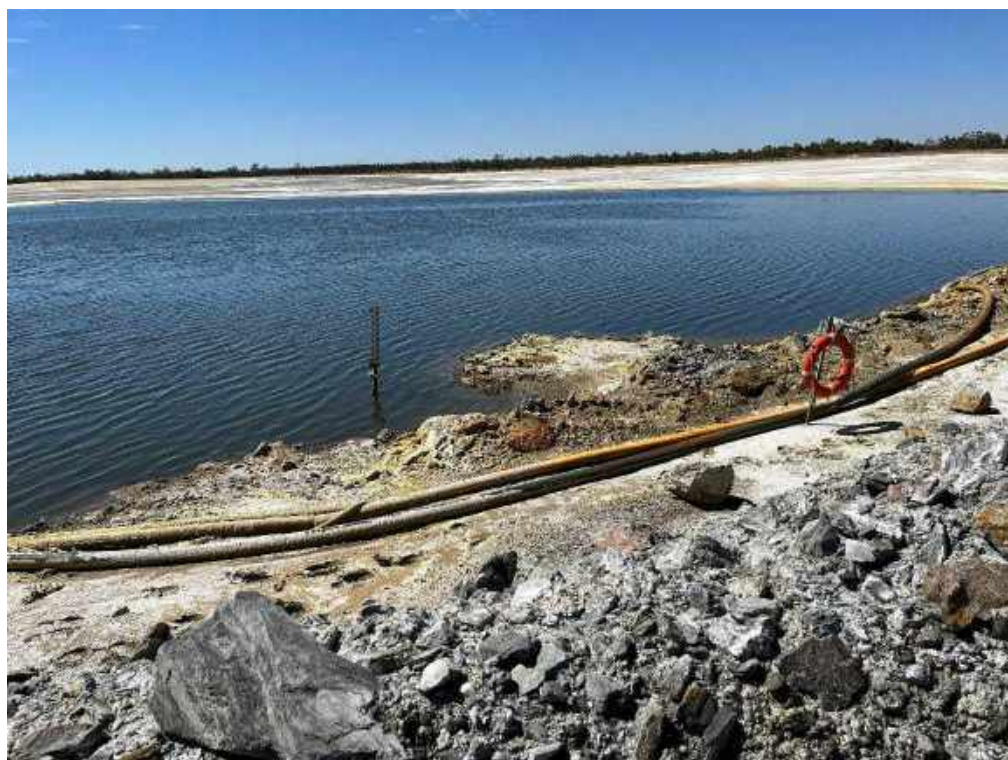
View of water level measuring staff and safety ring.
