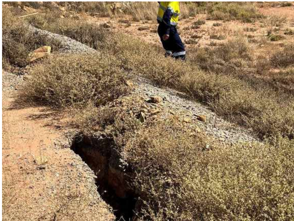
View of piping holes on intermediate berm, northern end.
