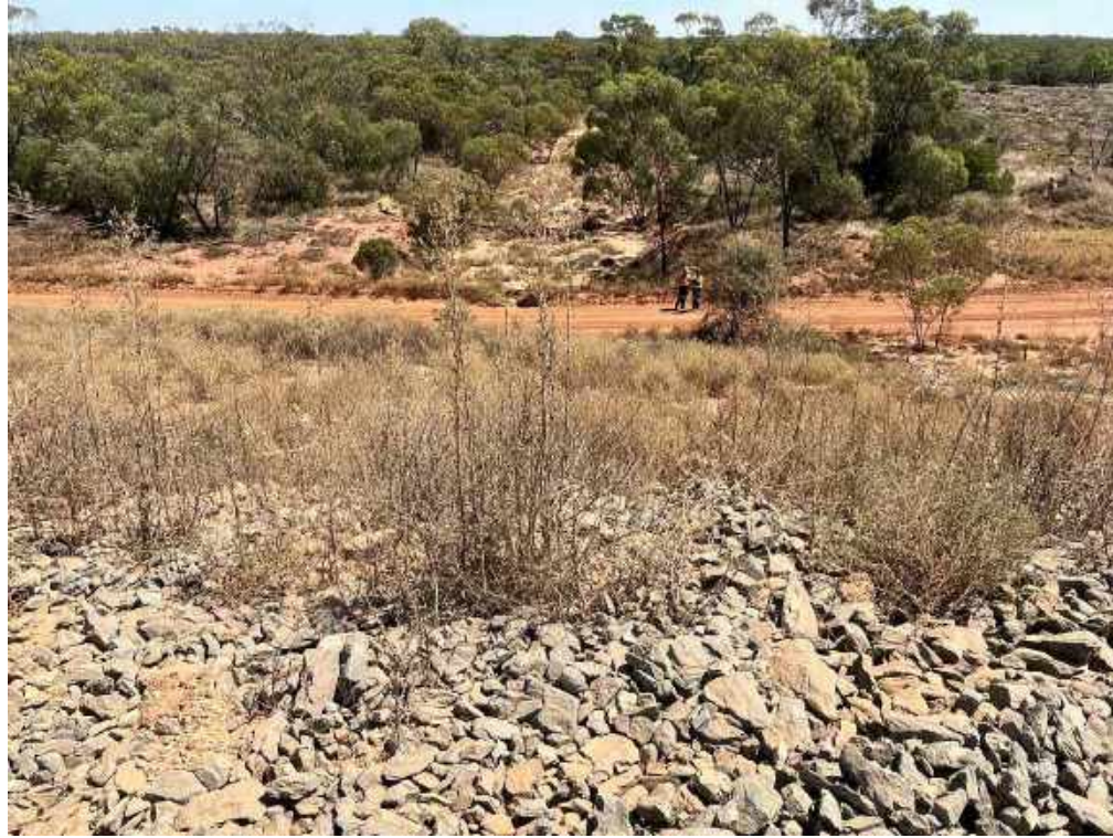
View looking downstream along spillway channel.
