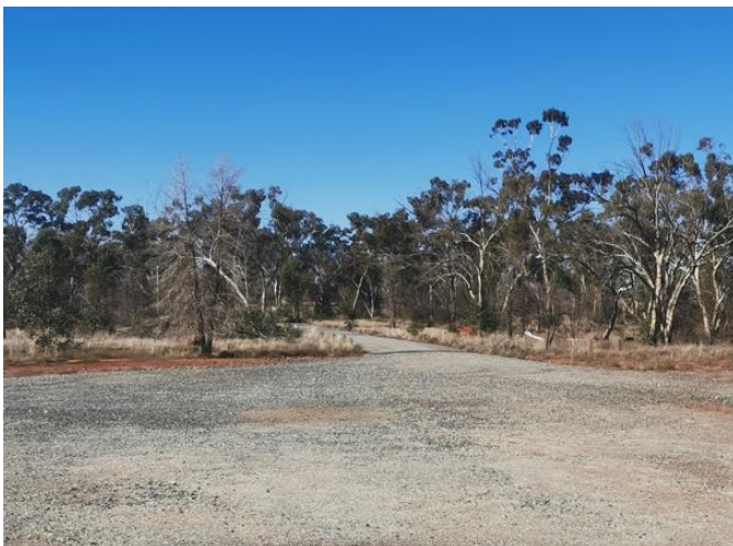
Photo 5 Access road and vent pad
