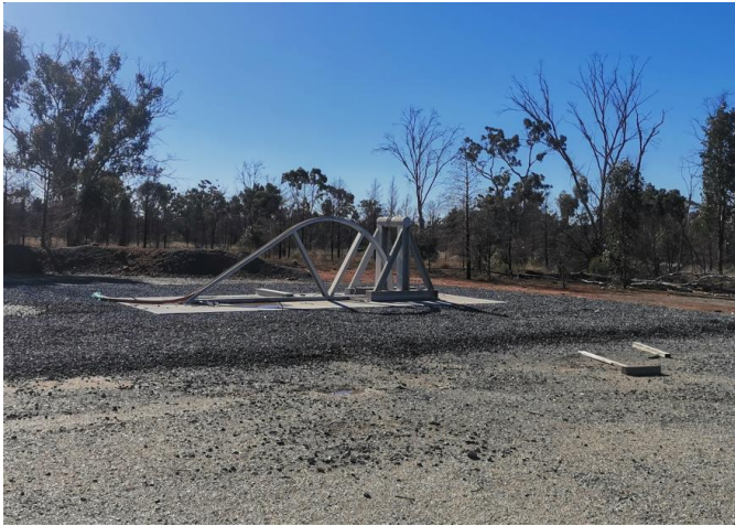
Photo 1 Vent under construction
