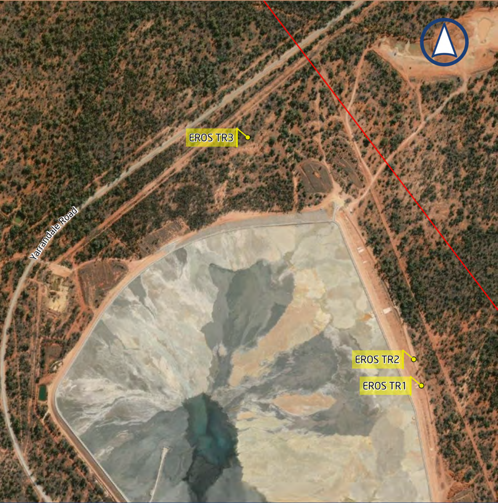
Figure 7 - Erosion Monitoring Locations
