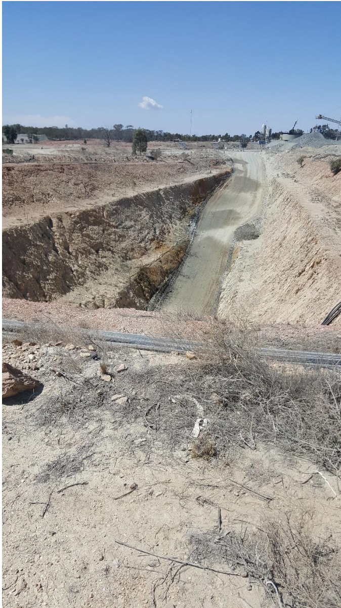
Dust control measures – entry to box cut
