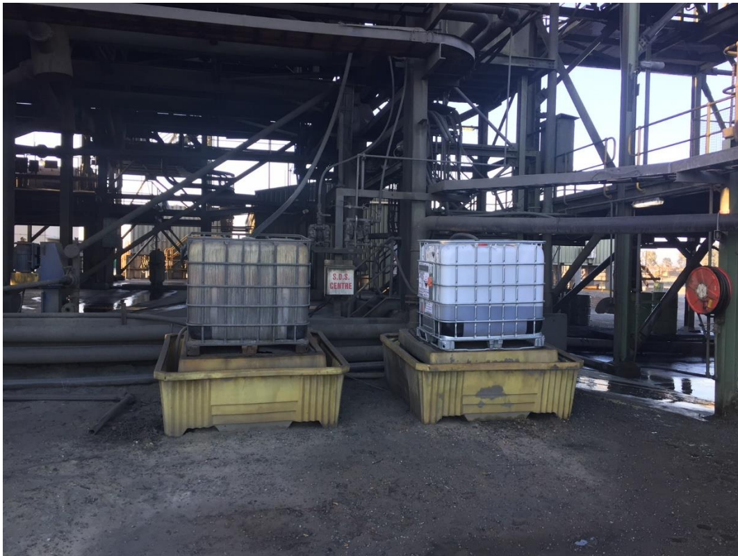
Workshop area (discolouration on ground is visible)
