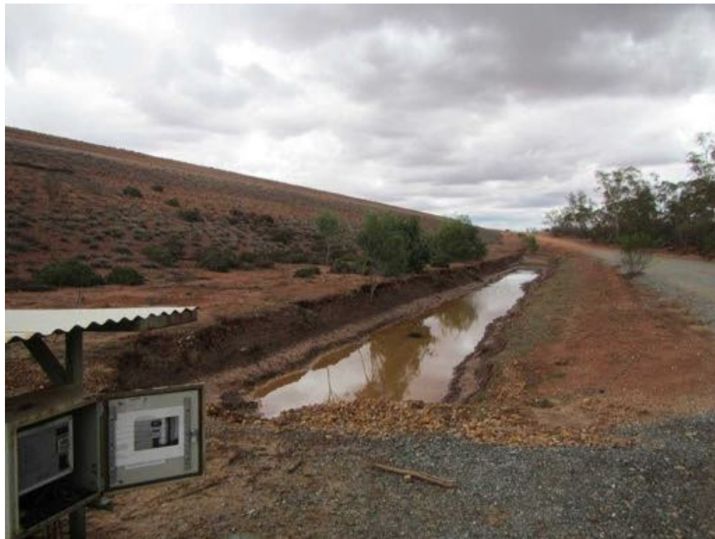
Downstream batter slope main embankment and downstream toe drain looking north.
