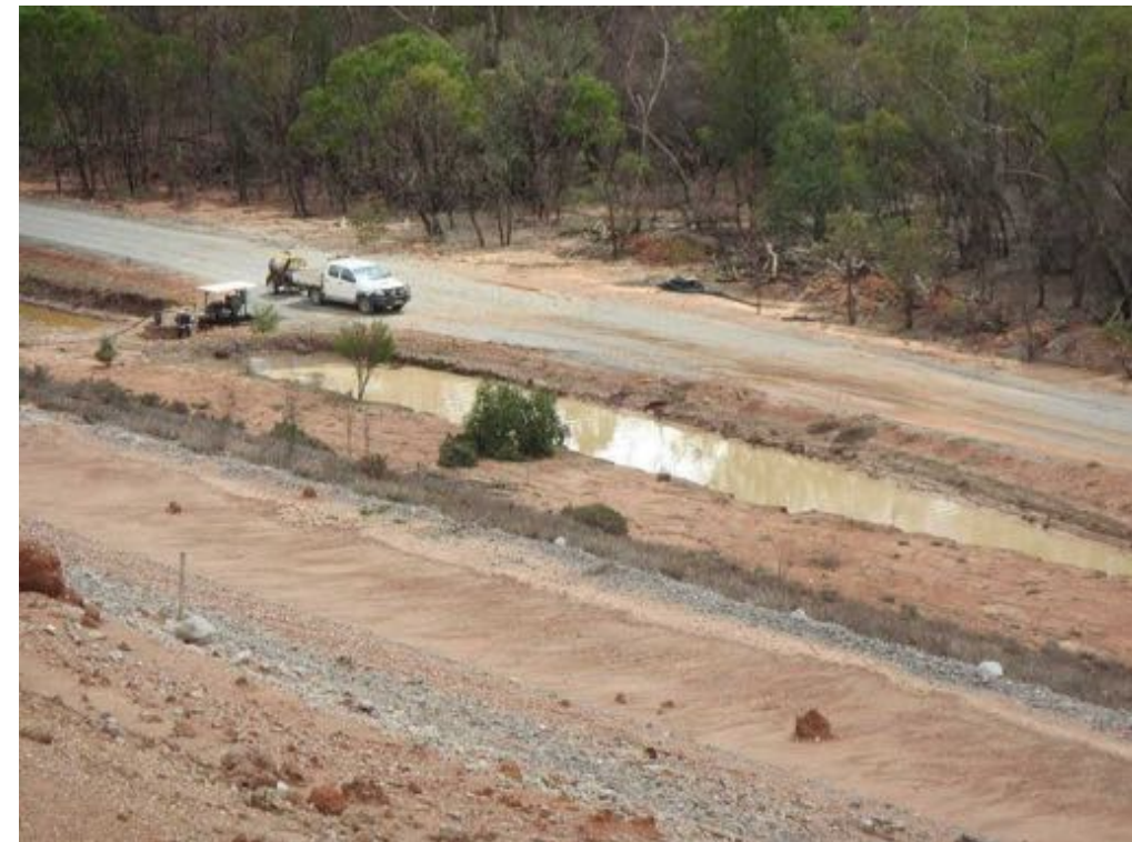
View of downstream sump. Recent rain in toe drains.
