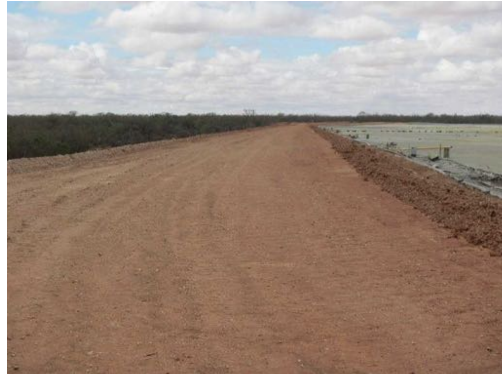
Looking south along main embankment crest.
