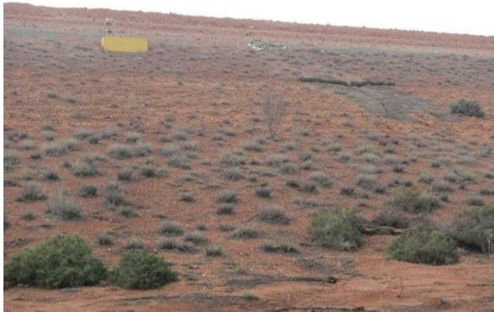
Main embankment batter slope with erosion protection, coir matting.
