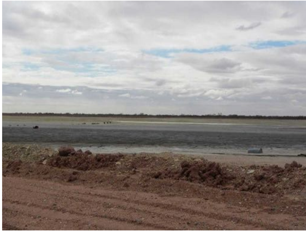
Looking east over tailings dam.
