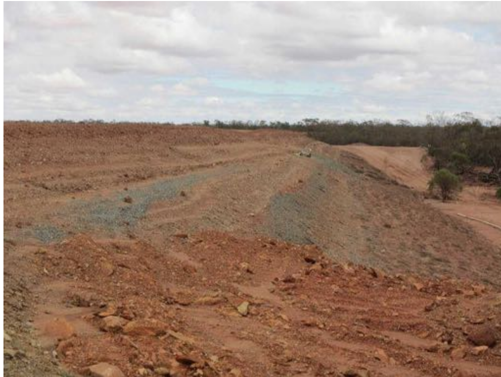
Northern embankment looking towards spillway area.
