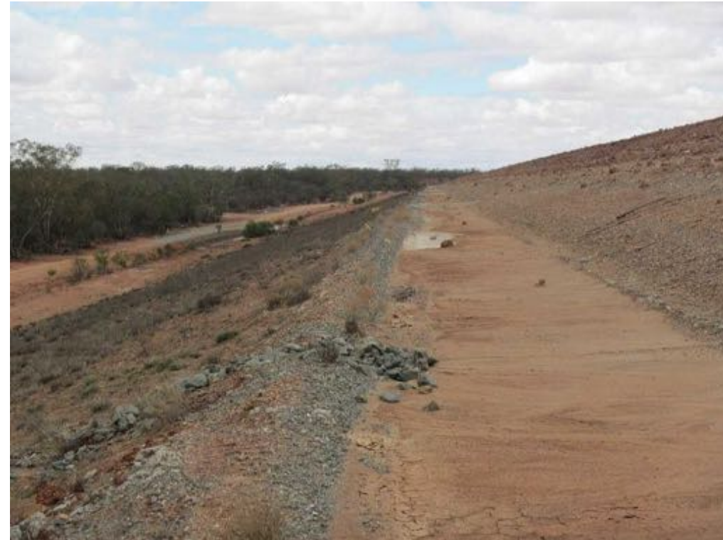
Intermediate berm main embankment looking south.
