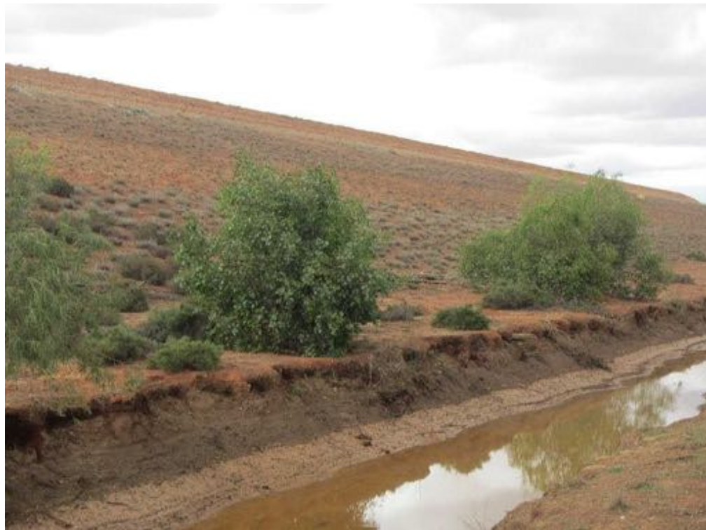
Small trees downstream of main embankment, not distressed.
