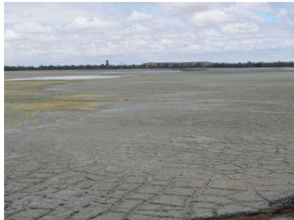
Looking across tailings dam from main embankment showing small decant pond.
