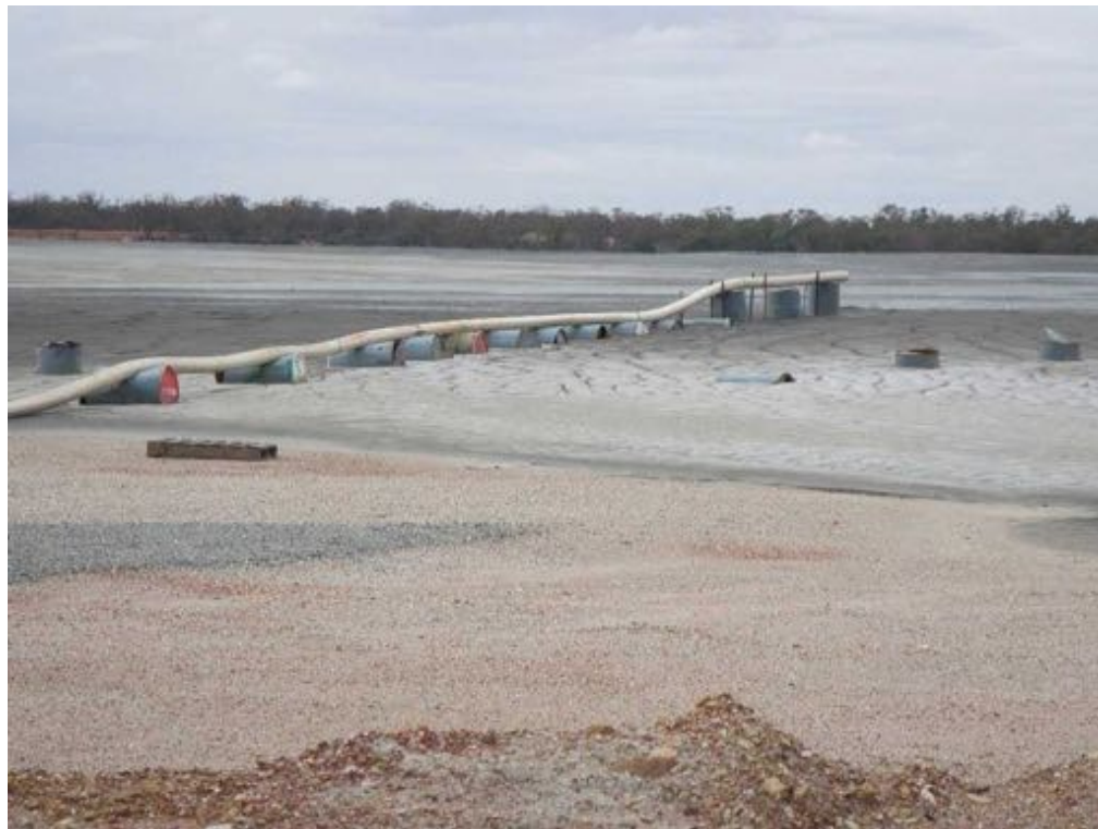
Extended spigot pipes supported on drums.
