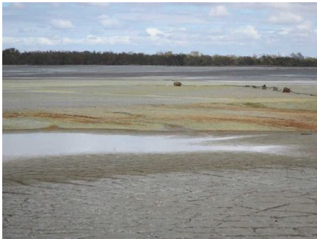
Downstream sump water discharge well out onto tailings beach.
