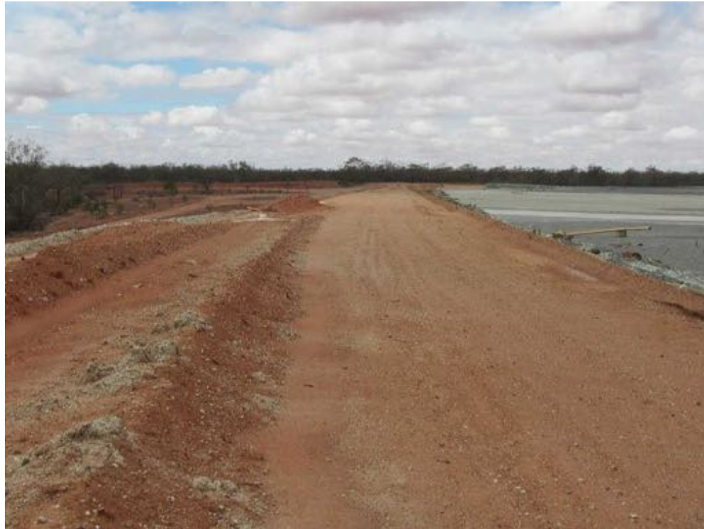
Main embankment looking south.
