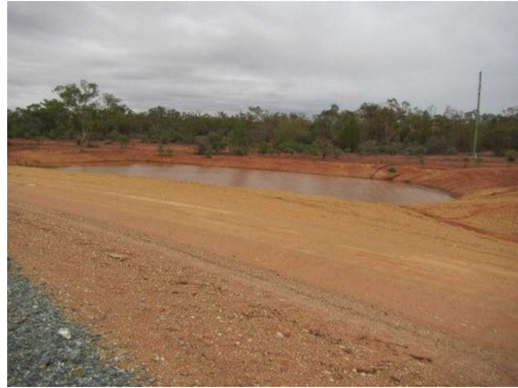
Sump downstream of western embankment used for construction purposes.
