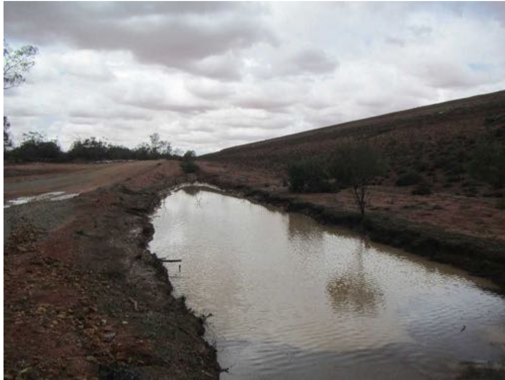
Downstream batter slope main embankment and downstream toe drain looking south.
