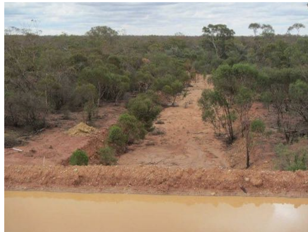
View along spillway channel. Recent rain on embankment.
